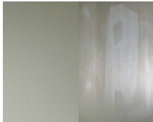
Figure 1. The touch-up problem. The left panel shows a section of a white, matte painted wall viewed straight-on. The right panel shows the same section of the wall viewed obliquely. Note the differences in surface lightness and gloss in the base and touched-up regions.
