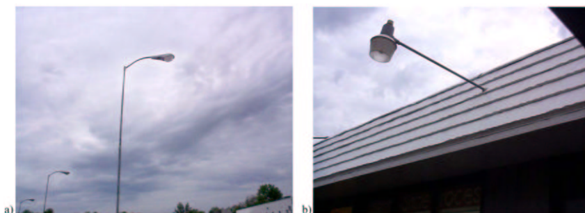
Figure 4: a) Mercury streetlight and b) mercury building light.
