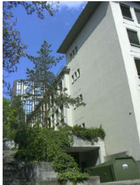
Figure 11. The back building hosts the Electronics Laboratory of the ETH
